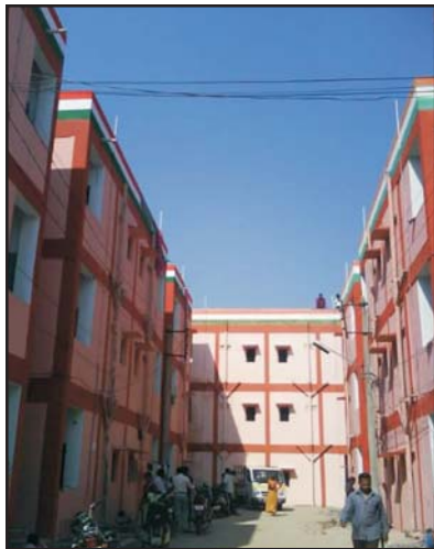
Fig.4 VAMBAY houses provided for rehabilitation of slum dwellers at Afzal Sagar
