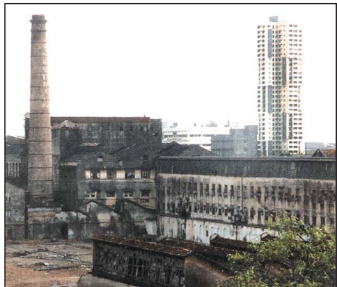
Fig. 5 Shree Ram Mills and a New High rise
