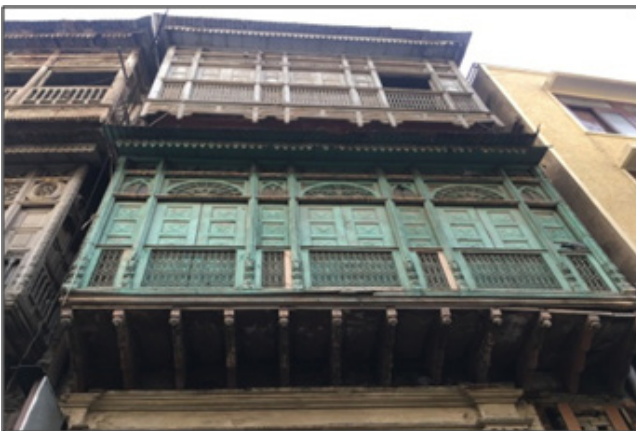
Figure 22 : Traditional Wooden Facades
