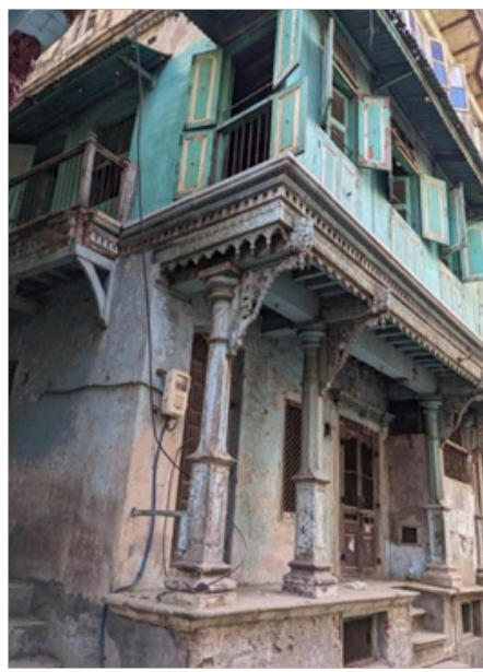
Figure 6 : Front Façade of a Pol Houses using Timber for Structural and Non-structural Members
