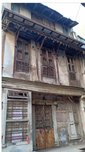
Figure 6 : Front Façade of a Pol Houses using Timber for Structural and Non-structural Members
